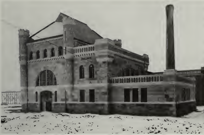
Calf Pasture pumping station, built in 1884. Boston Water and Sewer Commission.
